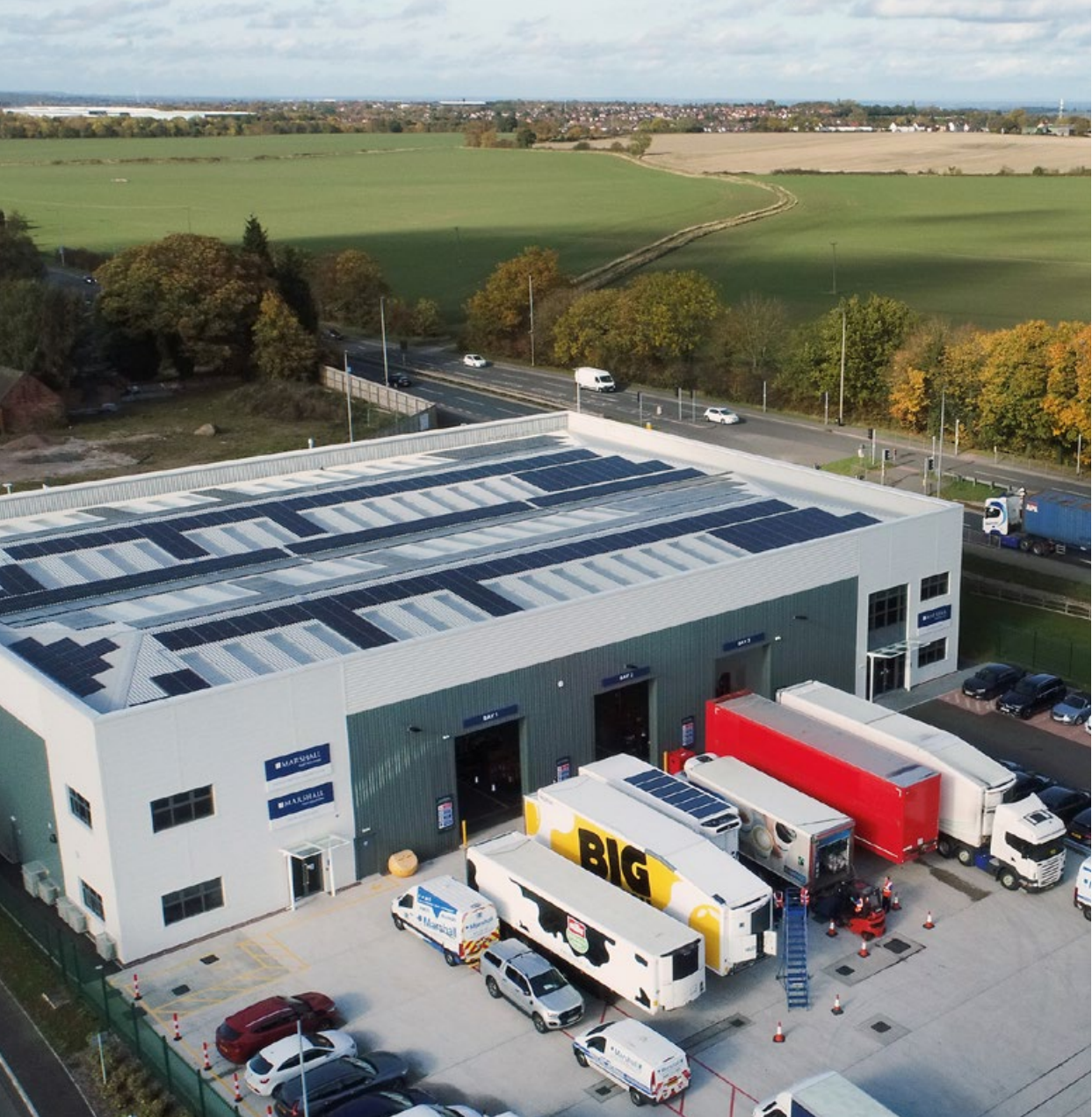
▼ Aerial View of Marshall Fleet Solutions Tamworth Super-Site
